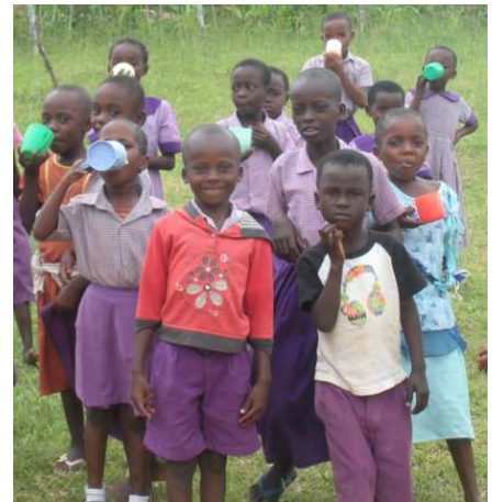
Upendo students enjoy morning porridge as they watch their school office being built.
